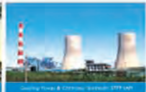
Cooling Tower & Chimney, Sector-13, Gurgaon, Haryana
